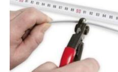
Define the sensor length from the standpipe height. Shorten the wire and Teflon hose to required length.
